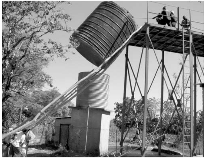
Water tanks at St. Theresa
